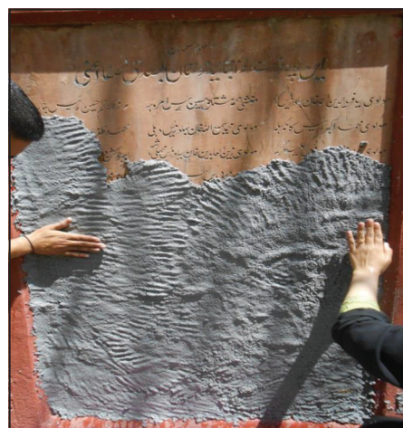
Figure 5: The removal of dust and dried salts with the help of nylon brush and applying of wet paper pulp on the object for the capillary suction.
