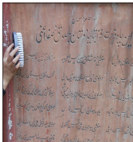
Figure 4: The removal of dust and dried salts with the help of nylon brush and applying of wet paper pulp on the object for the capillary suction.
